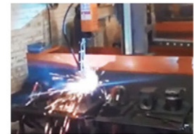
AUTO WELDING ROBOT
